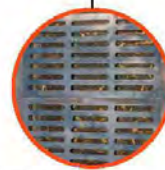
New drainage Heavy duty grated strip drain with heelsafe finish.
